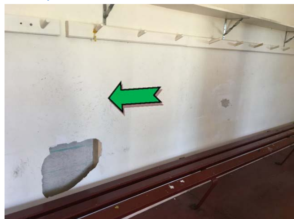
Photo 6. Interior, home change room, walls – non asbestos-containing fibre cement sheeting.
