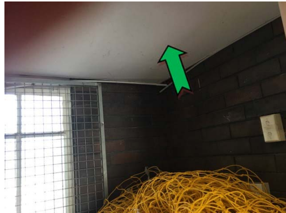
Photo 10. Interior, stores 1-4, lower ceiling – non asbestos-containing fibre cement sheeting.
