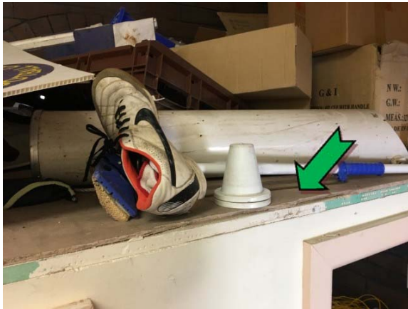
Photo 9. Interior, stores 1-4, upper ceiling – non asbestos-containing fibre cement sheeting.
