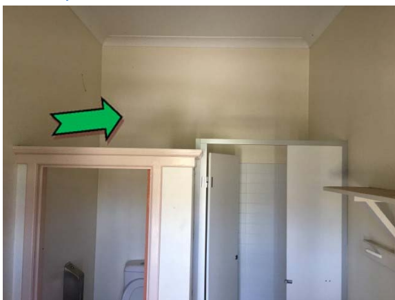
Photo 5. Interior, referee room, east elevation, wall – non asbestos-containing fibre cement sheeting.
