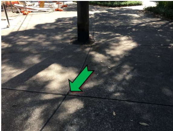
Photo 3. Exterior, east elevation, expansion joint – non asbestos-containing construction mastic.
