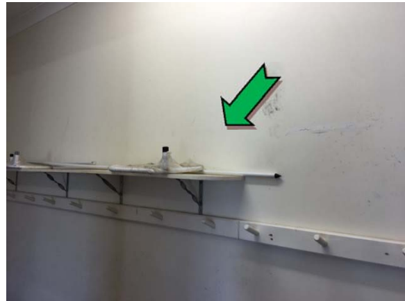
Photo 4. Interior, away change room, walls – non asbestos-containing fibre cement sheeting.
